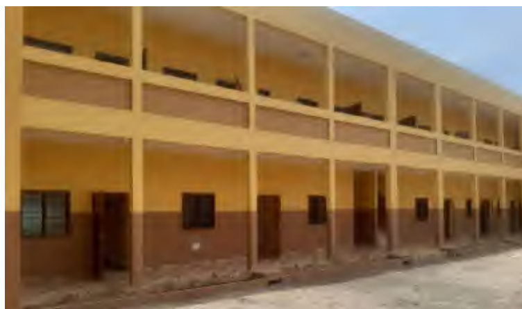
Construction is progressing according to plan, ensuring that the opening beginning of 2025 can take place.
